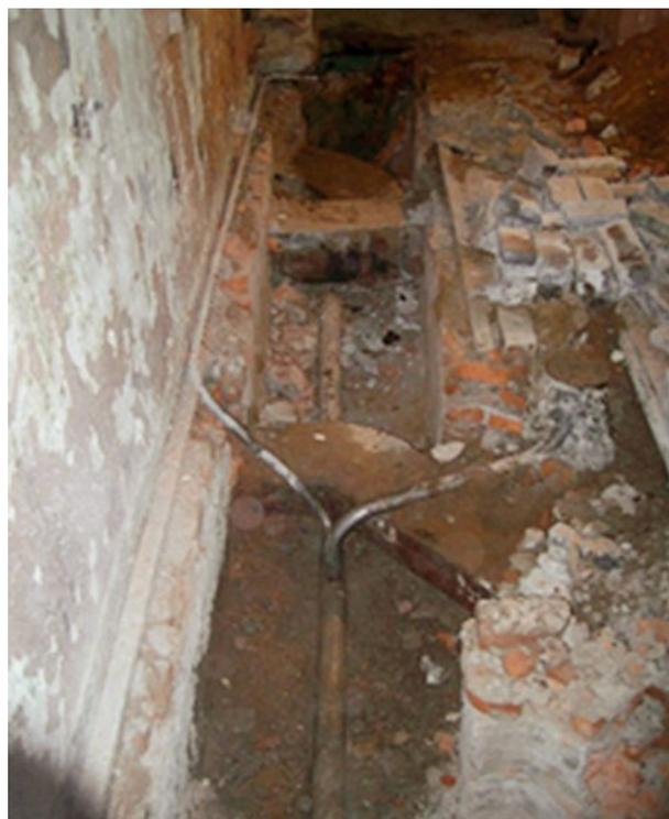
Fig. 5. Pipelines of abandoned special sewage system in compartment No. 49 of AST loop facility
