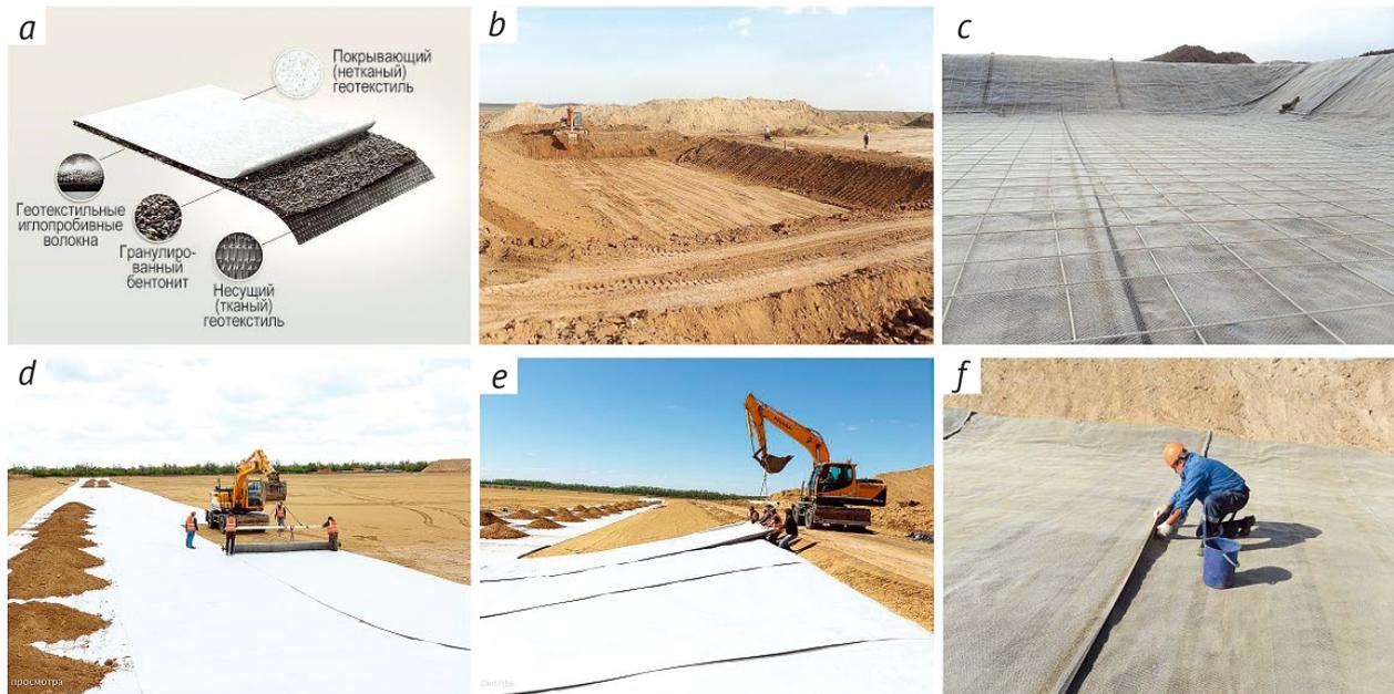
Figure 4. Layout of bentomat (a) examples of its application to ensure isolation of household waste landfills (before geotextile installation (b) after geotextile installation (c) examples of different layouts (d, e) and manual installation (f) during impervious barrier construction. Materials were presented by JSC Bentonite Company
