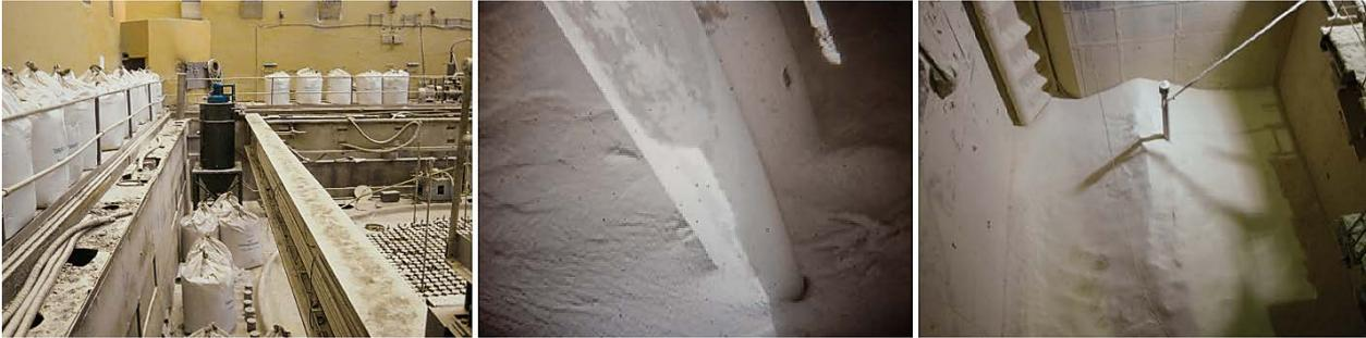
Figure 3. Construction of additional safety barriers inside PUGR EI-2 pit: the main hall during the backfilling process (left), barrier material inside the void spaces of the reactor pit (center), inspection channel inside the technological shaft (right)
