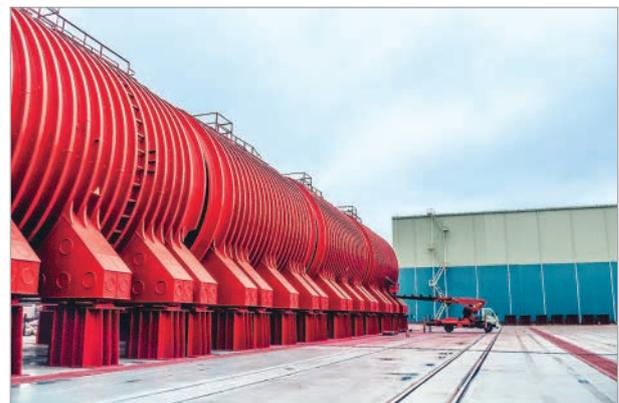
Figure 7. Emplacement of single-compartment reactor units into long-term storage facility
