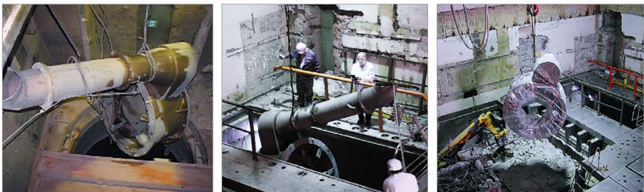
Figure 6. Staged dismantlement of reactor vessel's lower support
