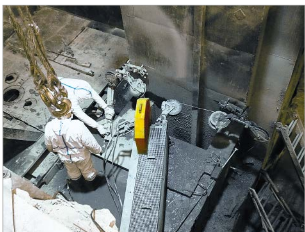
Figure 11. Layout of the dismantled part of MR reactor's shielding
