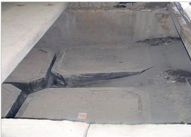
Figure 2. RW packages installed in DFRW compartment
