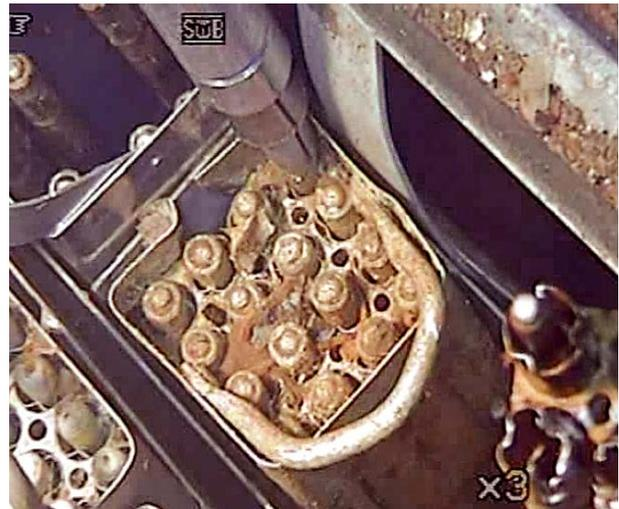
Figure 1. Retrieval of spent fuel elements from unconditioned SFAs under water using a purpose designed tool
