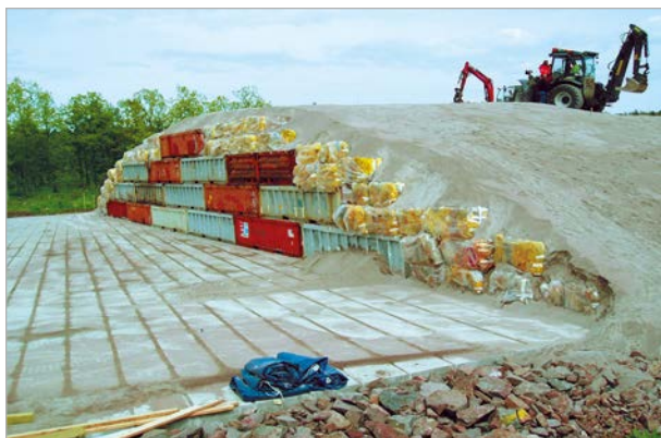
Figure 1. VLRW disposal method applied at the Oskarhamn NPP site (Sweden) during the construction of a covering cap [27]
