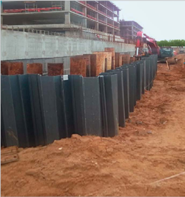
Figure 5. PVC sheet piling (construction of a facility in Skolkovo)
