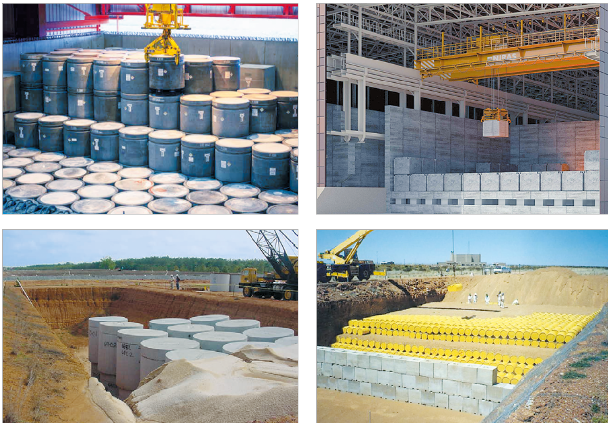
Figure 4. RW disposal in reinforced concrete RW packages with and without enclosing structures: top left – France [23]; top right – Belgium [24]; bottom left – USA, South Carolina [25]; bottom right – South Africa [26]
