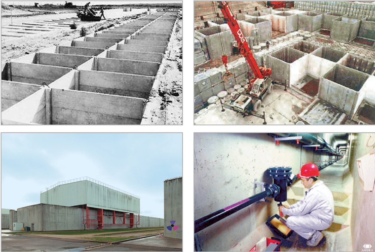
Figure 3. Evolution of RW disposal methods in France (top left: RW disposal in shallow trenches, 1969; top right: disposal on an above-ground concrete foundation without shelter structures, 1985; bottom left: modern surface RW disposal facility with concrete compartments, shelter structures, and inspection galleries for leak monitoring; bottom right: sampling operations in the inspection gallery) [16], [17]
