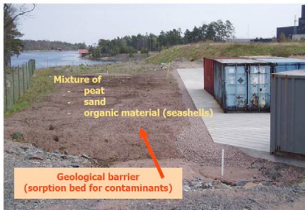
Figure 9. VLLW disposal facility at the Oskarshamn NPP, Sweden [31]
